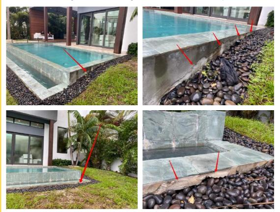
Recommend re-finishing exterior stucco siding around exterior barrier walls of pool. (Estimate: \$500 - \$1,000)
