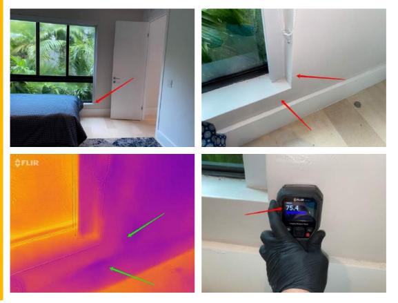
Recommend repairing or replacing water damage drywall around base of window. (Estimate: \$150 - \$250)
